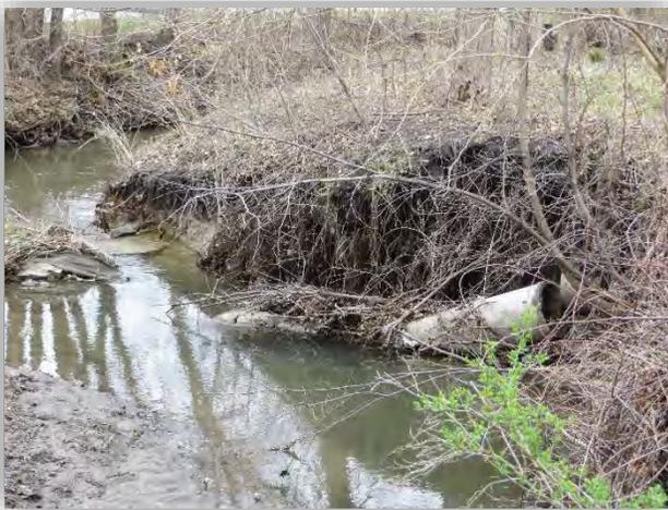
**Figure 2. Little Beaver Creek Storm Sewer Outlet Damage**
